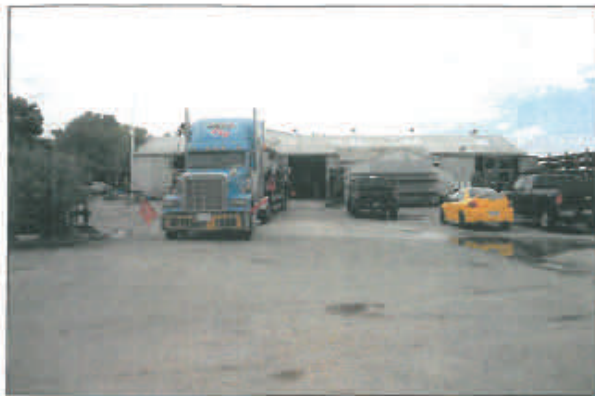
View of metal structures from north
