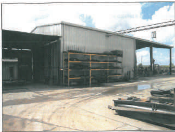
View of south structure
