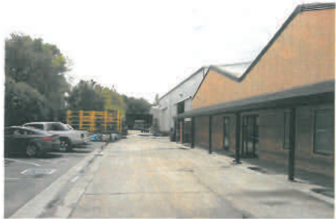
Buildings Looking South. River Road is to the Left of Frame.
