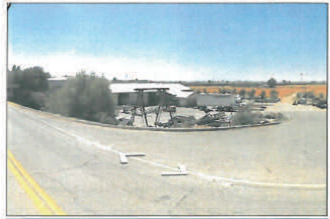
Subject as seen from River Road
